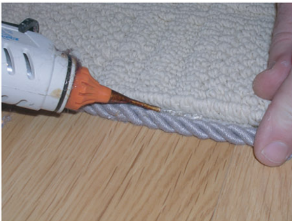
10) When you are happy with the join and corners etc, use the glue gun to apply a bead of glue between the binding and the carpet backing, pinching together as you go. Be careful not to get glue on the carpet.
