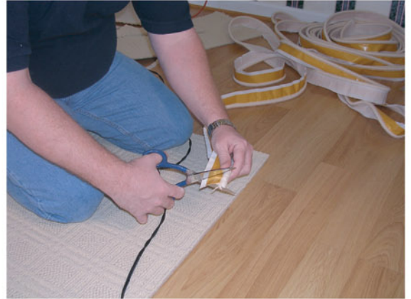
2) When Easybind is cut the rope part will fray, so apply Sellotape around the rope and cut through the middle of the tape.
