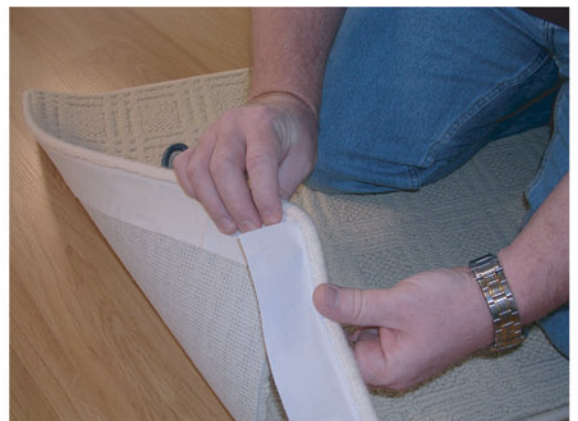
6) Corner technique shown from below the carpet.
